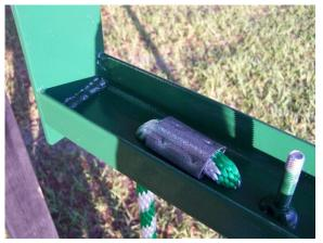
2. Pull the two rope ends until the flat side of the galvanized sleeve is near the inside bottom surface of the structural steel channel.
